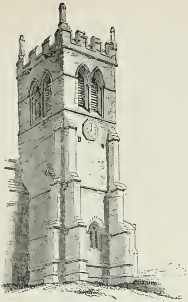
TOWER; RAVENSTHORPE, NORTHAMPTONSHIRE; c. 1300.
